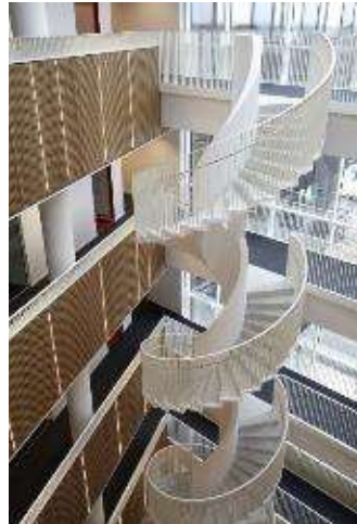
5. UHPC staircase in Per Aarsleff office building, Denmark
