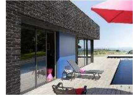
3. Artificial stone: Villa façade application, France
