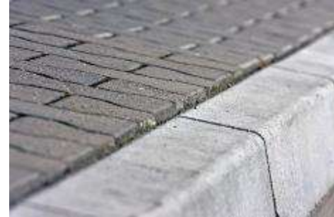
2. Paving blocks: Kerb, Poland
